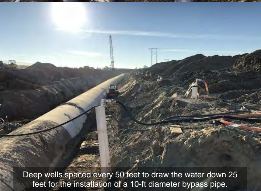
Deep well installation utilizing fully cased methods instead of drilling aids to keep the holes open to depth.
